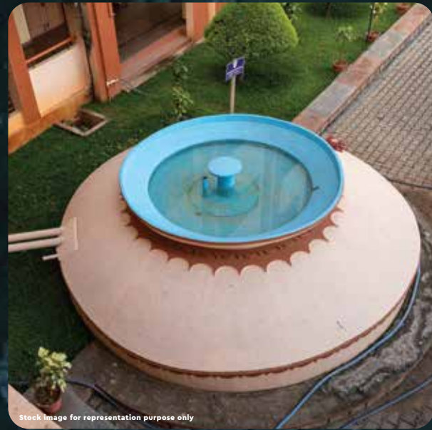
Rain harvesting system
