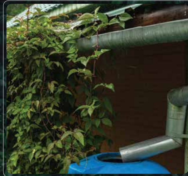
Smart V-shaped leveling of the parcel to direct water to collection points
